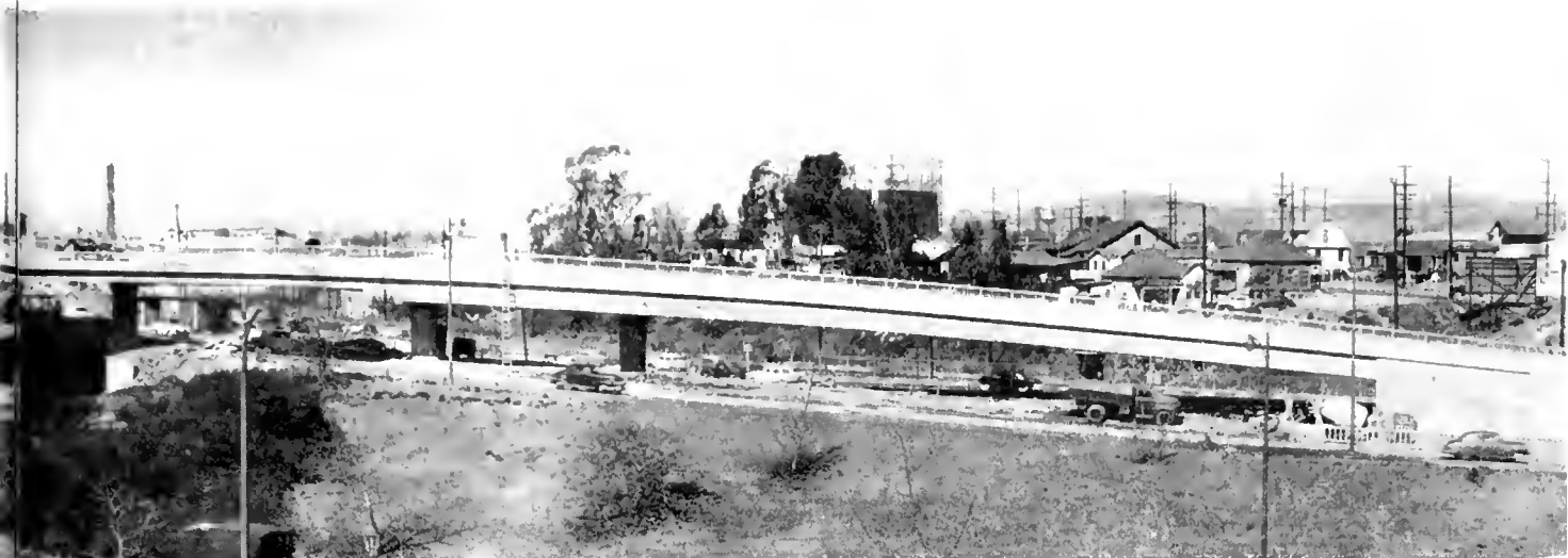
bridge showing the three levels of freeway separation at this point. Los Angeles City Hall in background.
